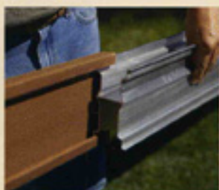
5. Slide bottom rail over the metal insert.*
