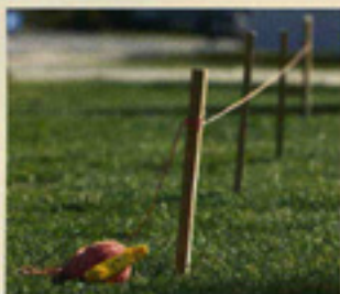
1. Stake out the fence line.
